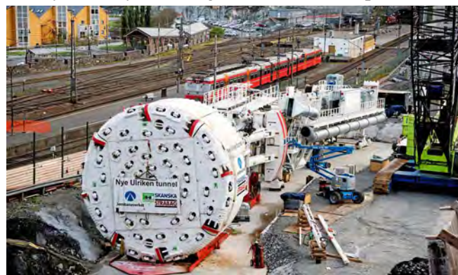
The colossal TBM
